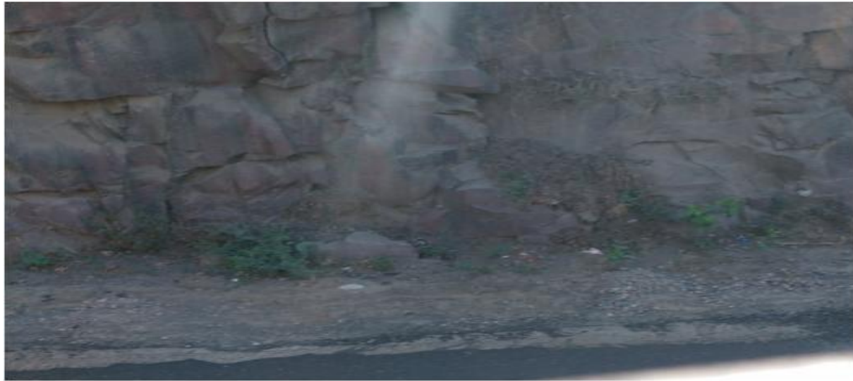
Figure. 4 Natural Hill along the Road Stretch.
