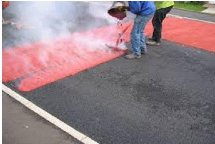
Application of the anti skidding surfacing to the pavement
