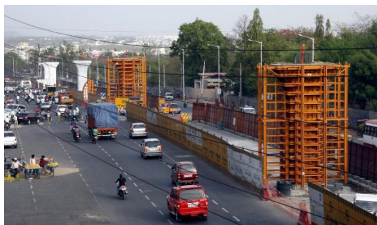
The roadway in between Uppal x road and Nagole
