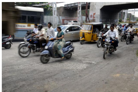
The roadway in between Taranaka and Lalapet
