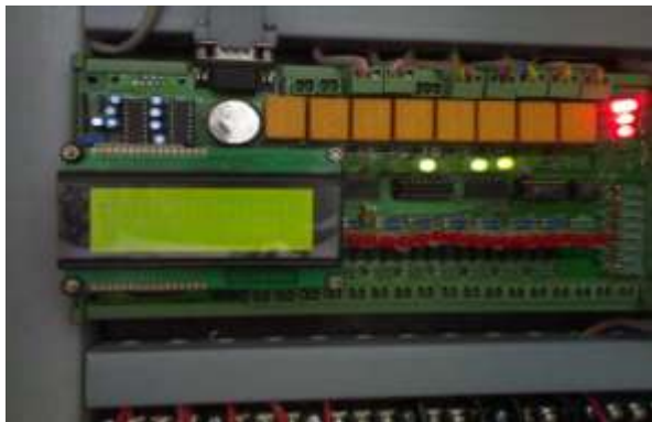
A Snapshot of DDC Controller in Operation with Relay on Board
