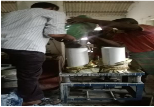
Fig 4: casting of CFT UPVC Tubes
